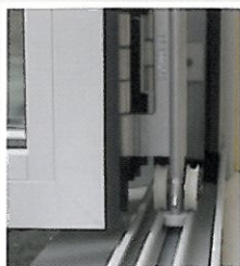
System SF70 running gear concealed between door panels
